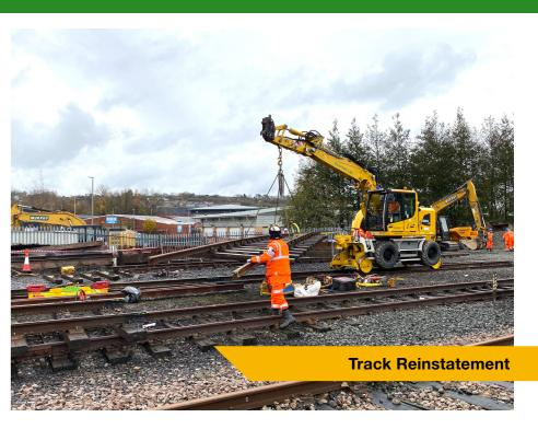
Following the track reinstatement, top ballast was installed in advance of a tamper passing through.
