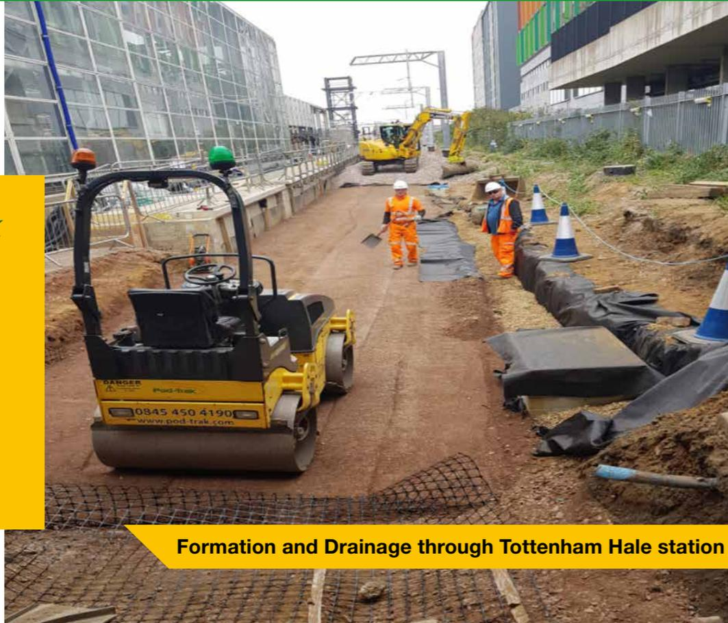
*Pod-Trak undertook the construction of 5.5km of track foundation and bottom ballast as well as over 2km of track drainage.*
