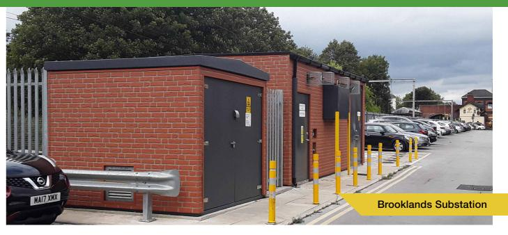
To cope with the electrical demands of increased traffic on both the Altrincham and Bury lines, a new substation was built on each line to provide additional power for the Trams.
