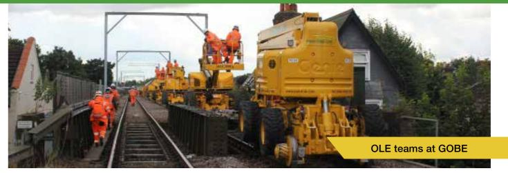
Pod-Trak undertook the electrification of the Eastern half of the Gospel Oak to Barking route on behalf of Balfour Beatty. The electrification of the lines was undertaken by Network Rail as part of their London Railway Upgrade Plan which doubles the capacity on the line and improves the air quality of those who live and work near the railway.
