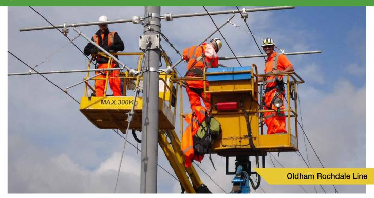
Co to install all of the overhead line equipment (OLE) including Traction Power on the Phase 3 extensions to the Manchester Metrolink.
